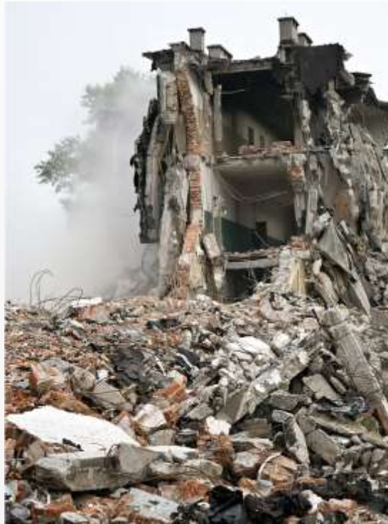
拆除（砖混）垃圾
